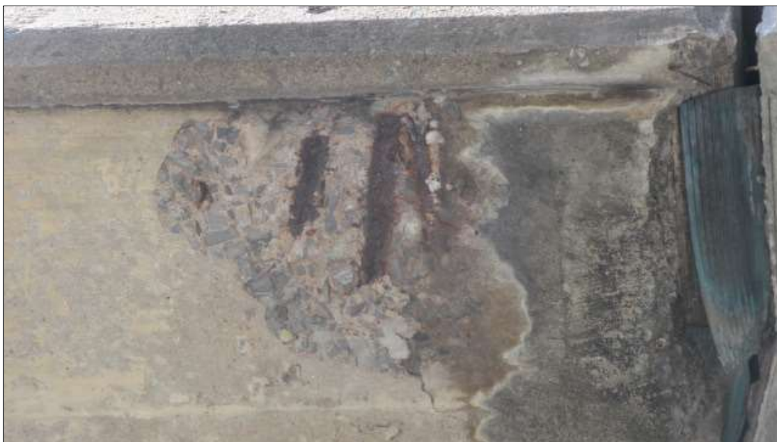
Span 1 Deck: 2 Square Feet of Exposed Rebar: Present without measurable section loss. 8" diam. popout under the lt. o'hang above bent 1 cap with rebar exposed.
