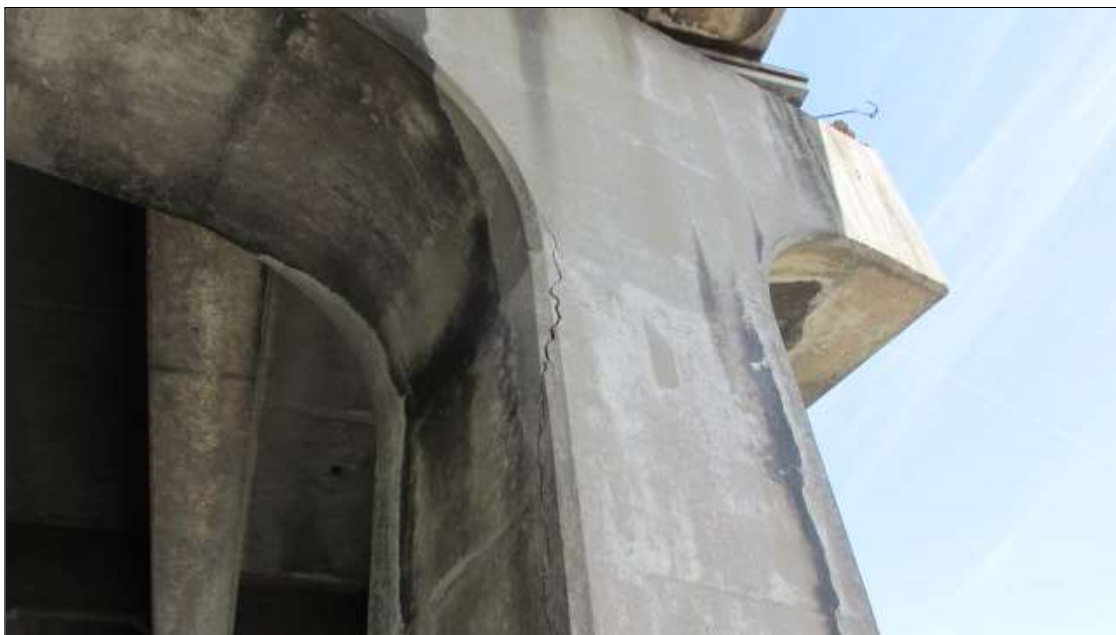
Bent 2 Pile 1: 1 Each of Cracking (RC and Other): Width 0.012-0.05 in. or spacing or 1.0-3.0 ft. vertical cracking on the east face for 9'
