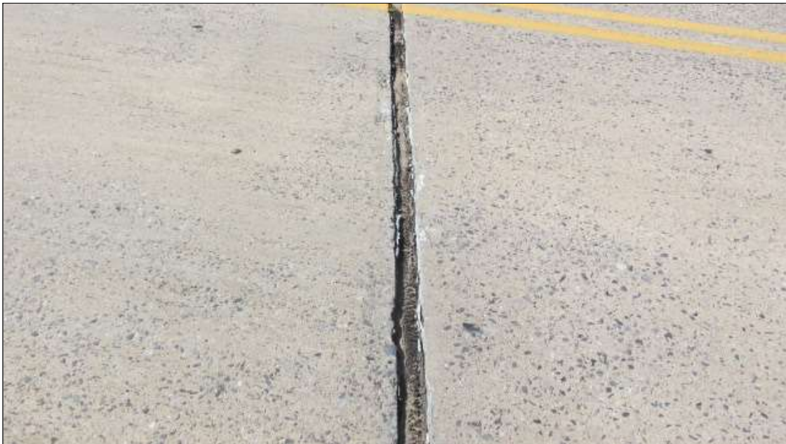
Expansion Joint 3 : 40 Feet of Debris Impaction: No debris to a shallow cover of loose debris may be evident but does not affect the performance of the joint.
