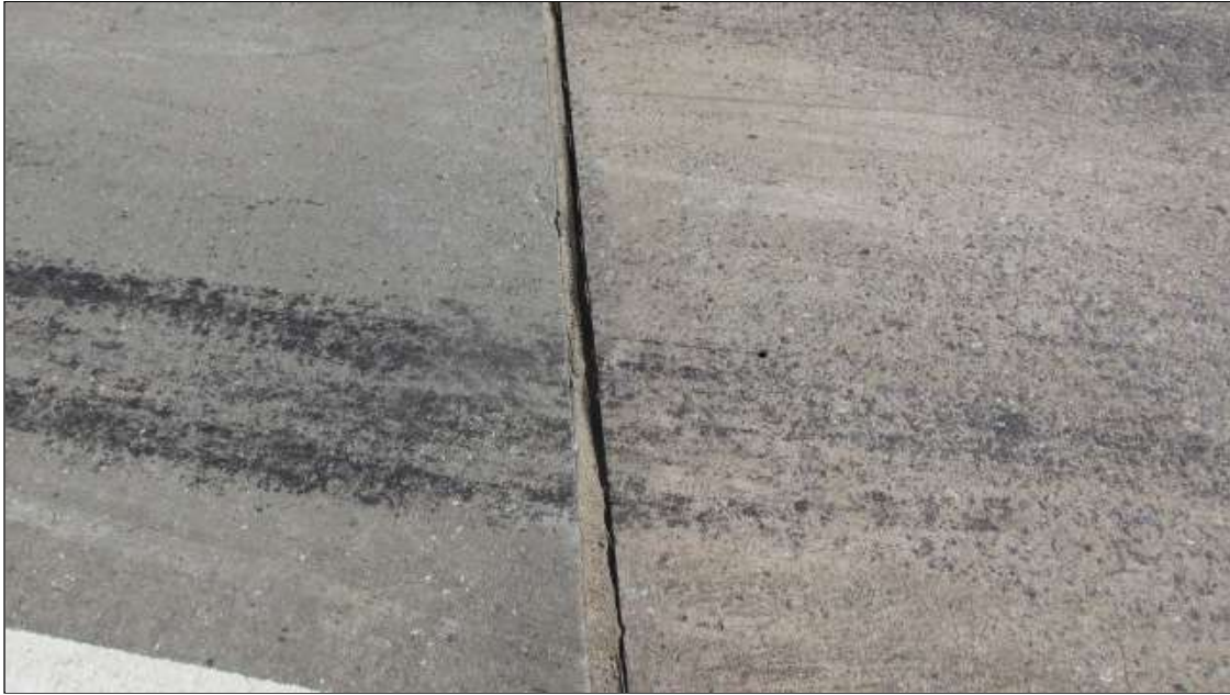
Expansion Joint 2 : 40 Feet of Debris Impaction: No debris to a shallow cover of loose debris may be evident but does not affect the performance of the joint.
