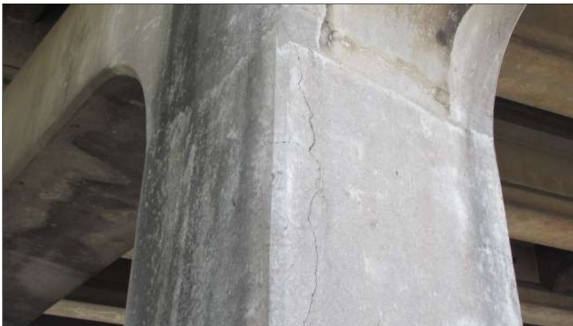
Bent 2 Pile 3: 1 Each of Cracking (RC and Other): Width greater than 0.05 in. or spacing of less than 1 ft. vertical crack runs 8'
