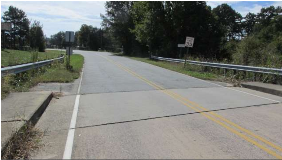
guardrail looking east
