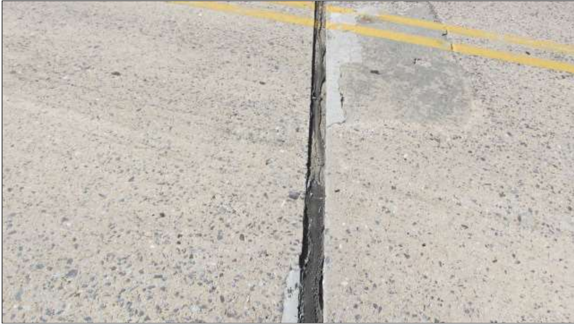
Expansion Joint 1 : 40 Feet of Debris Impaction: No debris to a shallow cover of loose debris may be evident but does not affect the performance of the joint.
