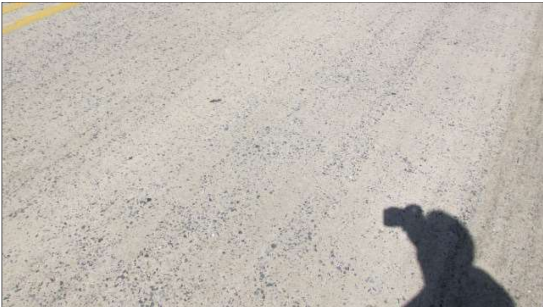
Span 4 Deck: 2000 Square Feet of Abrasion/Wear (PSC/RC): Abrasion or wearing has exposed coarse aggregate but the aggregate remains secure in the concrete.
