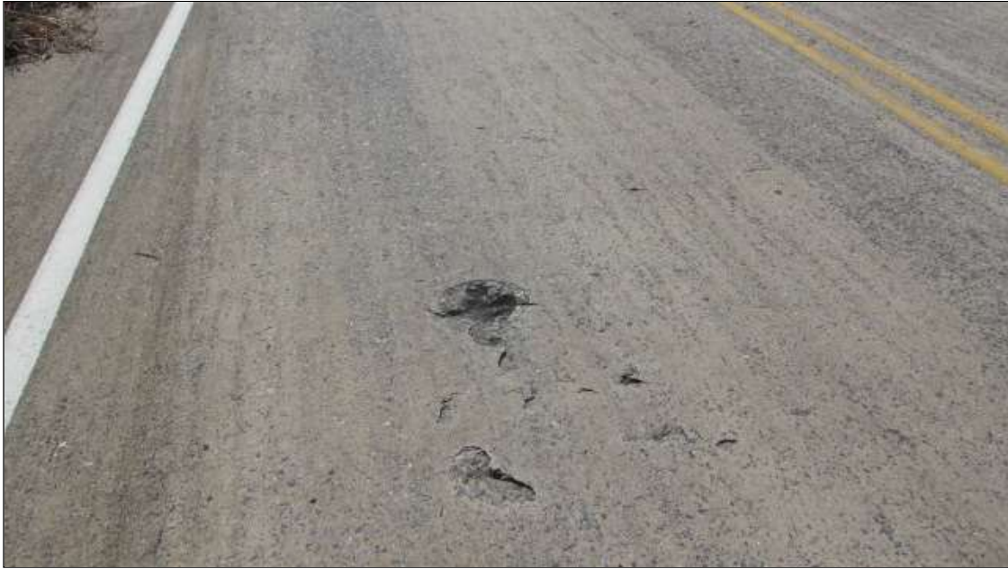
Span 3 Deck: 2 Square Feet of Delamination/Spall/Patched Area: Spall greater than 1 in. deep or greater than 6 in. in diameter. Patched area that is unsound or showing distress. Does not warrant structural review.
