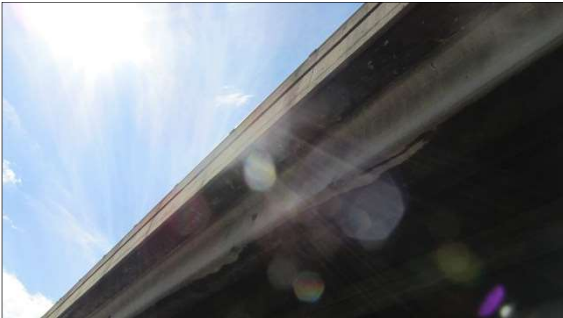
Span 2 Beam 1: 2 Feet of Delamination/Spall/Patched Area: Spall greater than 1 in. deep or greater than 6 in. diameter. Patched area that is unsound or showing distress. Does not warrant structural review. chip spall due to impact from vehicle 2' along the bottom corner over rt. lane looking south
