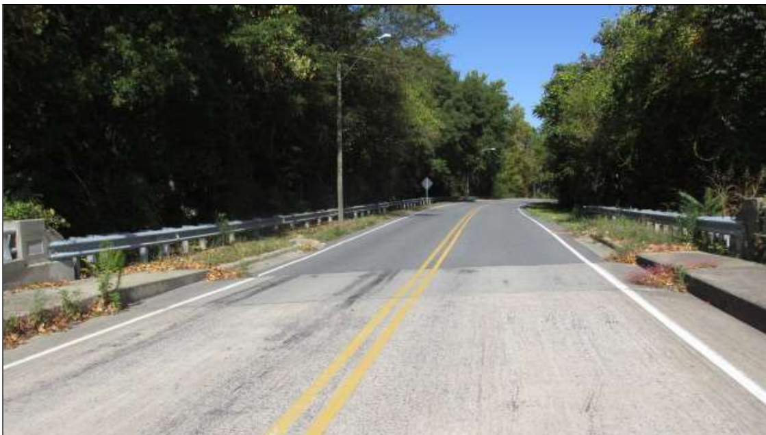
guardrail looking west
