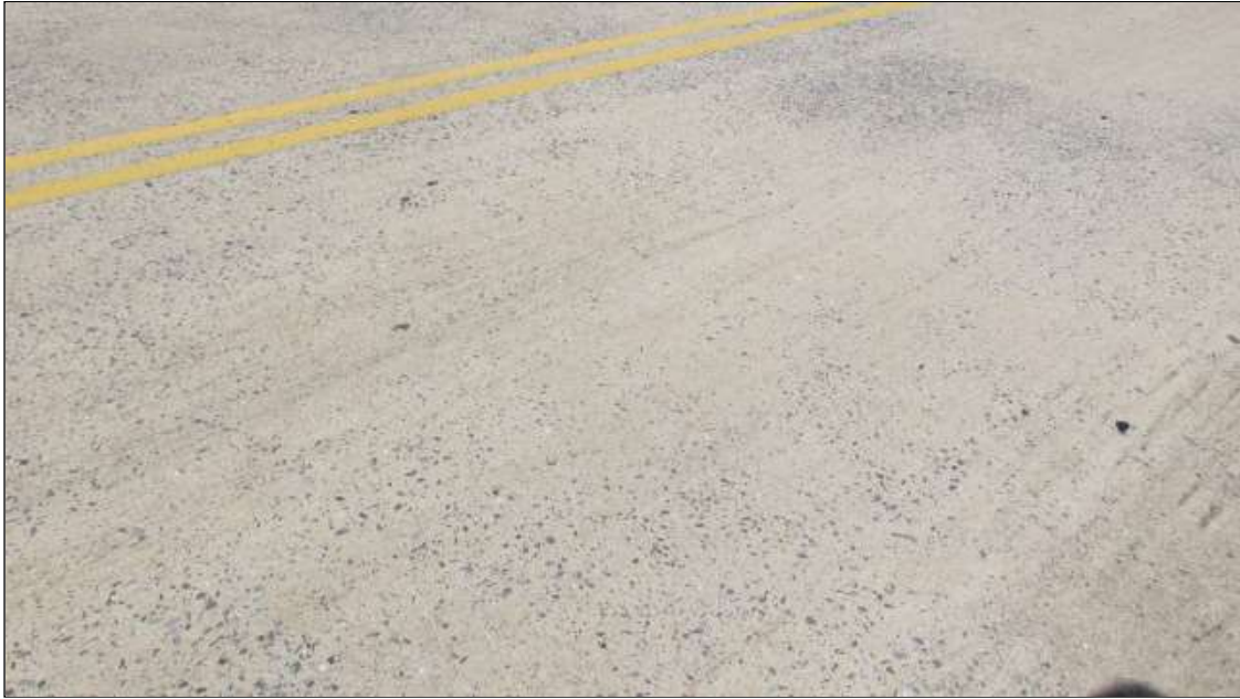
Span 2 Deck: 2000 Square Feet of Cracking (RC and Other): Width 0.012-0.05 in. or spacing of 1.0-3.0 ft.
