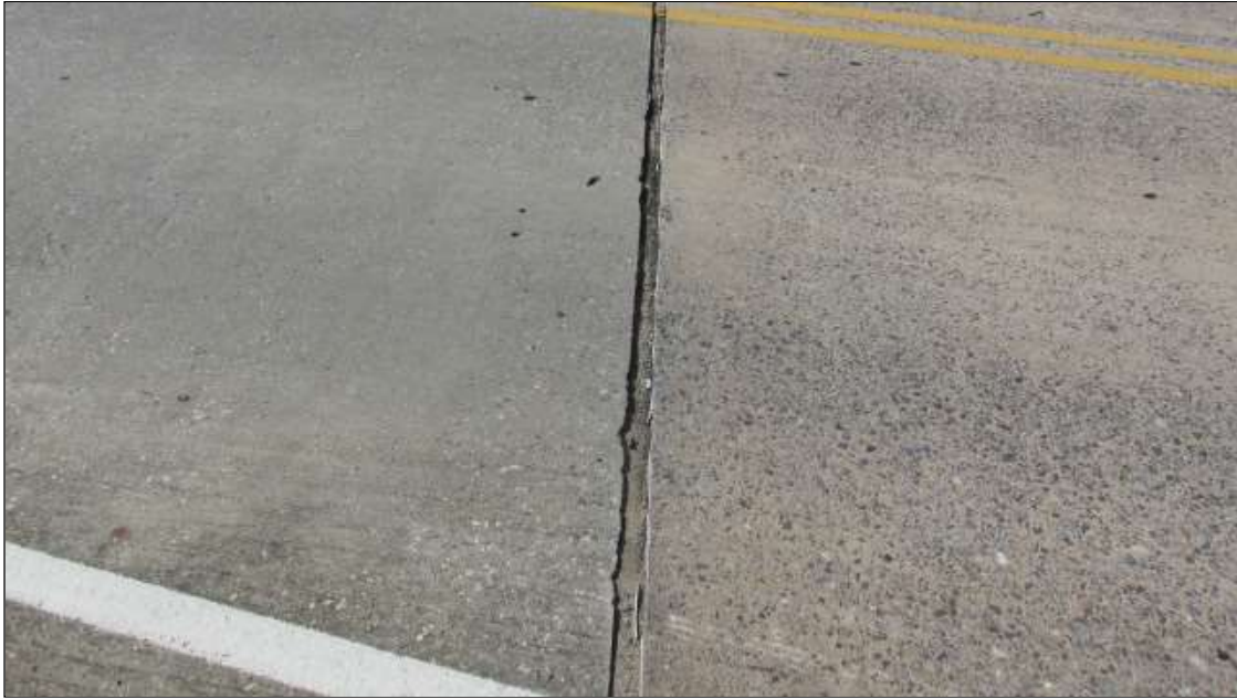
Expansion Joint 5 : 40 Feet of Debris Impaction: No debris to a shallow cover of loose debris may be evident but does not affect the performance of the joint.
