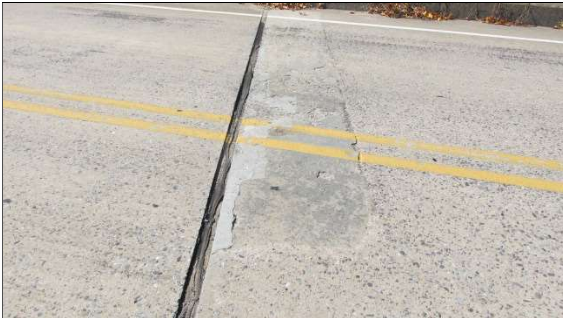
Span 1 Deck: 20 Square Feet of Delamination/Spall/Patched Area: Delaminated. Spall 1 in. or less deep or 6 in. or less in diameter. Patched area that is sound. concrete patch 2' l x 10'l in the rt. lane at the east end of span 1 at joint.
