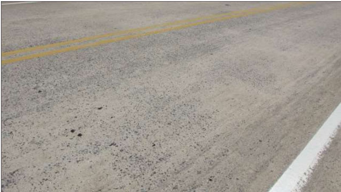
Span 1 Deck: 2000 Square Feet of Cracking (RC and Other): Width 0.012-0.05 in. or spacing of 1.0-3.0 ft.
