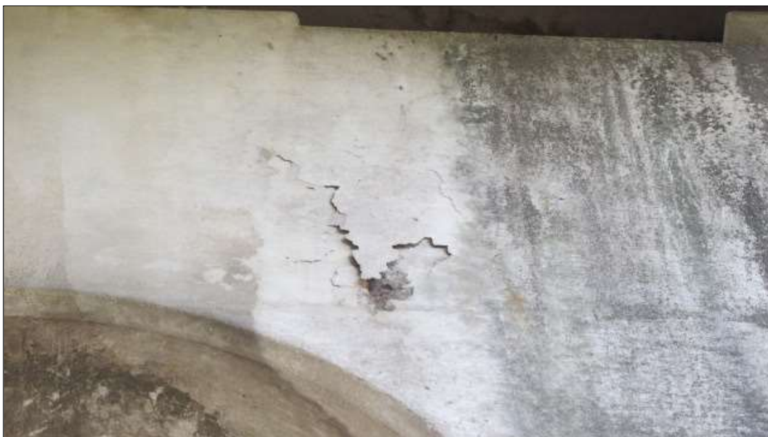
Bent 3 Cap : 1 Feet of Cracking (RC and Other): Width 0.012-0.05 in. or spacing of 1.0-3.0 ft. 1' diam. crack/spall in progress on the east face of the cap in bay 1.
